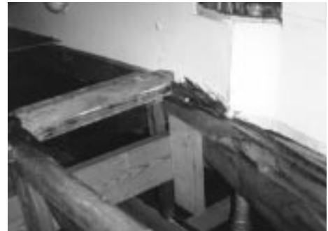
Floor structure of Trades Building
